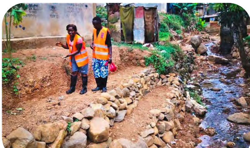
Trained community volunteers banking and constructing gabion at Dwarzack communities. © UN Sierra Leone
